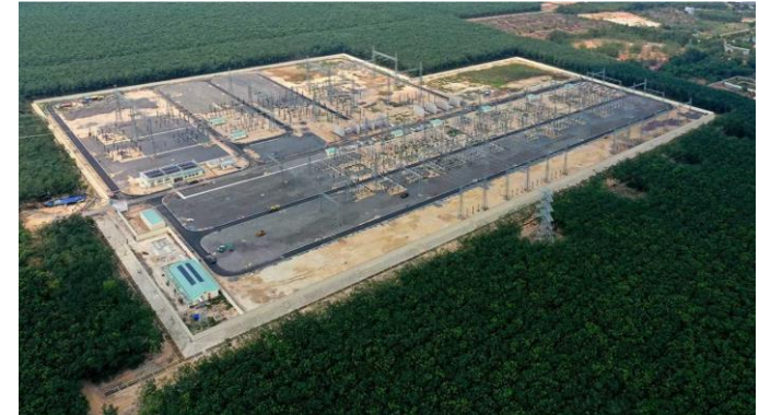
Project: Long Thanh 500Kv Station Client: ATS JSC Content: Deluge Valve
