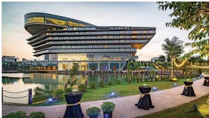
Project: Marriott Ha Noi Client: BITECO Content: Valves
